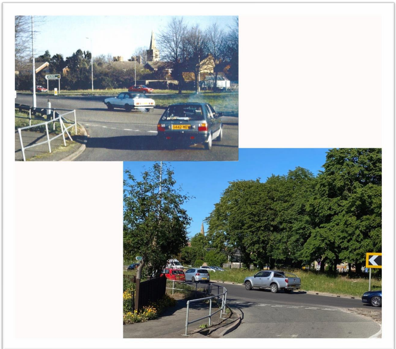
FIGURE 49 PICTURE 6 - BUCKDEN ROUNDABOUT
